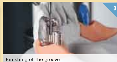
Finishing of the groove
